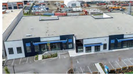
47,506 SF Industrial Building CARPENTER STREET 2138 Carpenter Street, Abbotsford, BC
