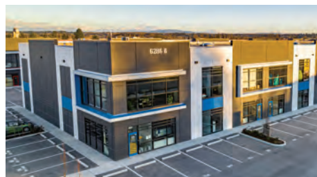
119,887 SF Over Three Buildings WESMONT CENTRE 6286 203rd Street, Langley, BC
